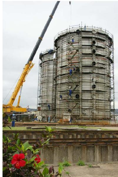
The two converters took Metso ND a total of 65 000 man-hours to complete - all of which were successfully completed injury free. By December 2008 both converters - each weighing 395t, with individual shipping envelopes of 17.8 m by 15.5 m by 24.6 m in height - was ready for shipment.
