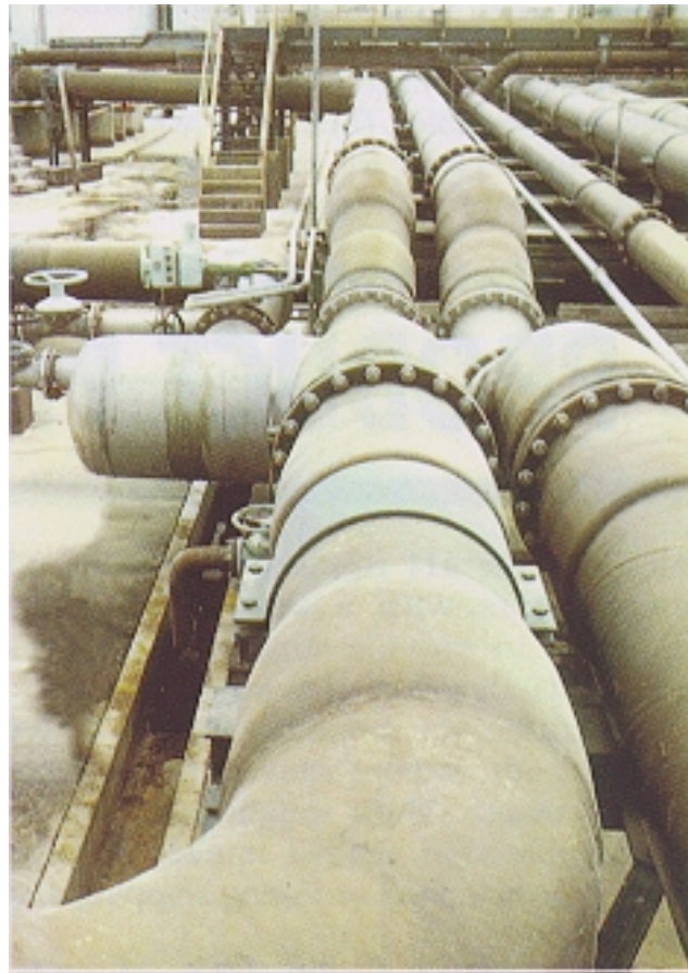
Figure 19. Abrasion Resistant Pipe for Phosphate Fertilizer Process Slurry
