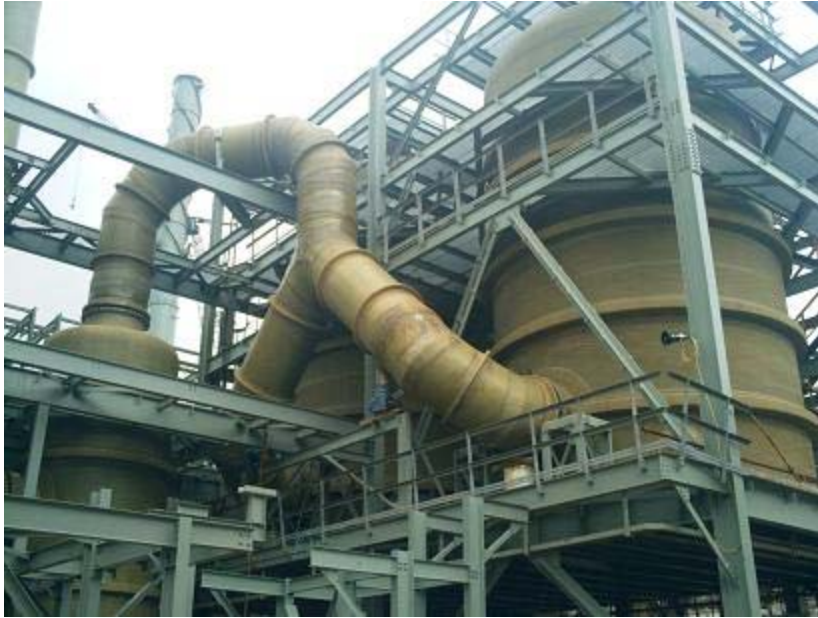
Figure 6. Dual wet gas mist eliminator vessels for a spent acid regeneration plant under construction.
