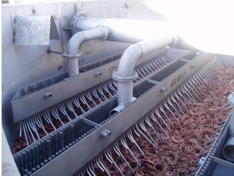
Following installation of the upper section of the tower, the distributor was supported by hangers, leveled and the topping-off of packing was completed.
