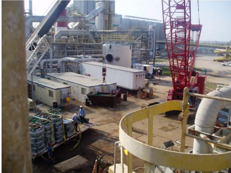
Reconstruction of the HRS tower allowed loading of the packing before the top was placed on the tower. The first layer of packing was hand placed using notches in the packing wings to support a highly open interface between the packing and the support grid. Saddles, locked in place in this manner, are capable of supporting manpower without incurring damage. Random dumping of green boxes was carried out from this point until the tower packing was completed.
