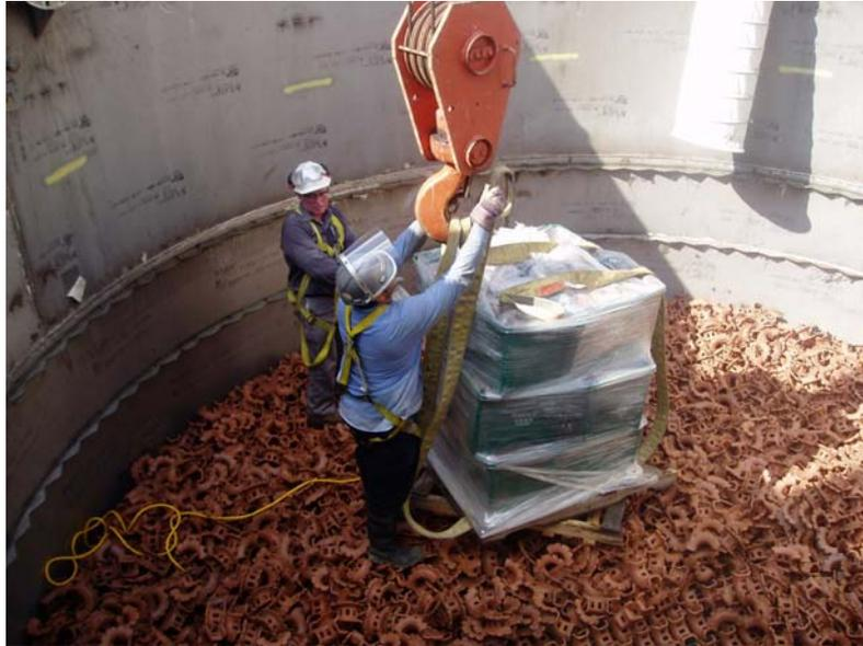
A wall layer of 2 inch standard saddles was placed to create a high wall pressure drop in the lower part of the tower forcing the gas away from the wall and into the HP+ packing. Metal deflectors, seen in the photo, had been installed in the new shell that could have precluded the need for the 2 inch saddles.
