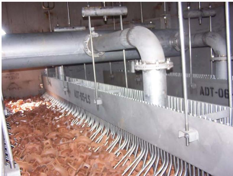
Clean-up of the tower below the packing support level consisted of removal of chips and broken saddles created during removal of the previous packing. Only several small pieces of red shale were found.
