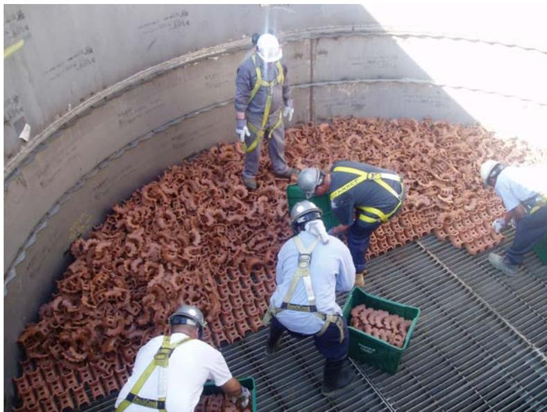
As well, with the top removed from the tower entire pallets were hoisted into the tower and placed on top of packing already in place to allow the work crews to unload the new pallet. No plywood or any other protective device was needed to protect the packing and no damage to the packing occurred.
