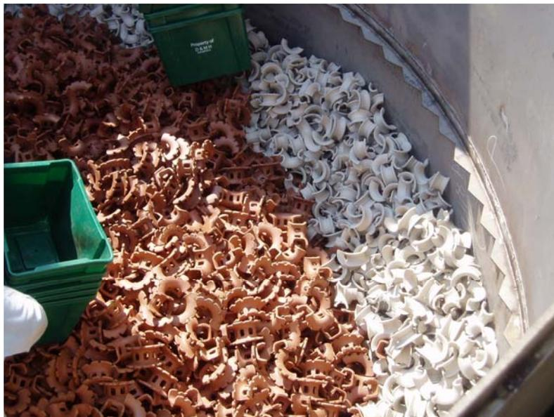
Prior to topping-off the packing, the distributor was placed in position resting on the packing with no need for plywood or other protection to the packing. No damage to the packing occurred.
