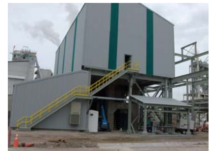
From Piles to Building: Installation of the TG-3 Building
