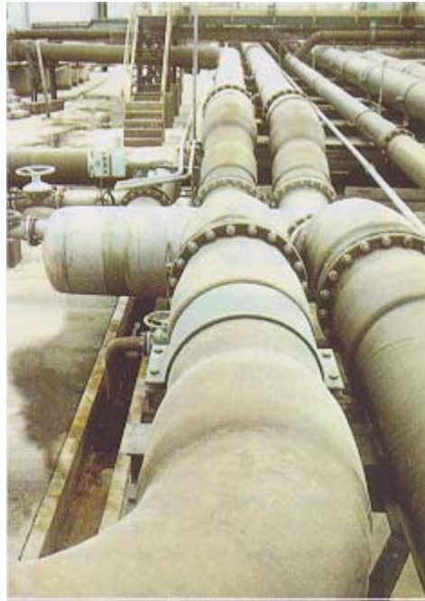
Figure 8. Abrasion Resistant FRP Pipe for Phosphate Fertilizer Process Slurry
