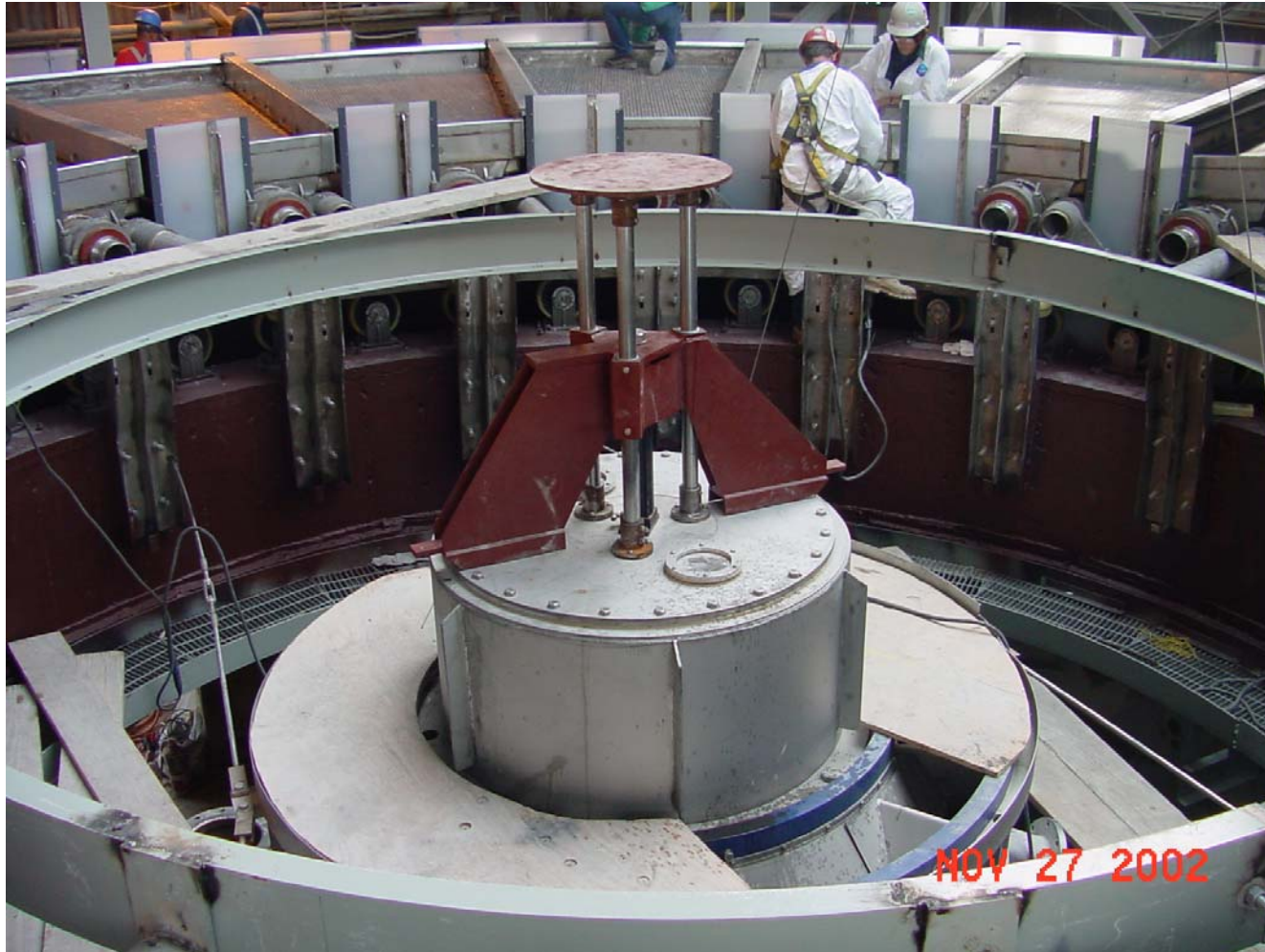
BAC valve (patented) with hydraulic lift for the manifold.
