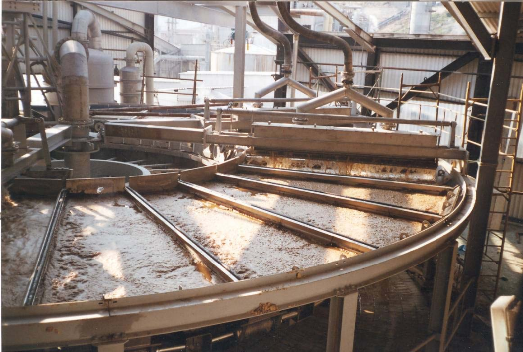
24-75 TDI Prayon filter in operation at PFI Kavala since July 2003.
