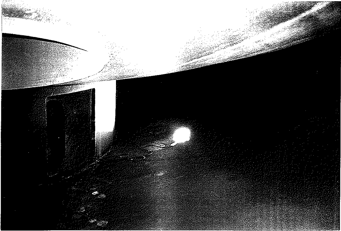
Figure1 Typical Appearance of Bed No. 1 Outlet
